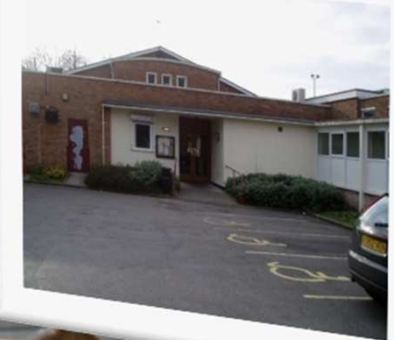
Banks Leisure Centre
