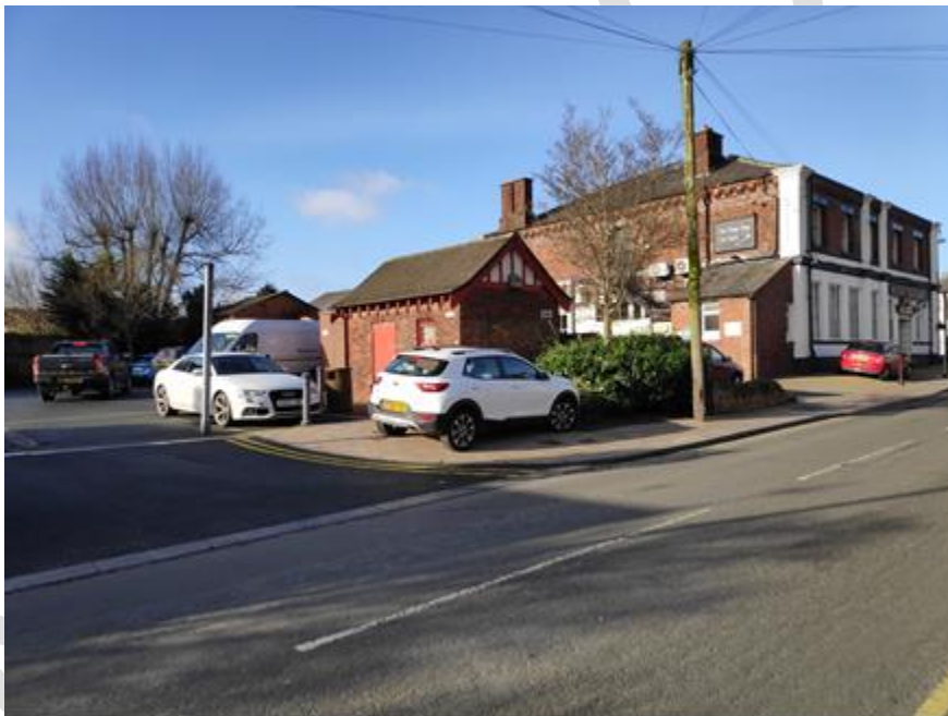
Gents & Wheelchair Toilet
